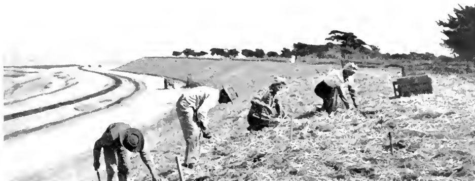
Planting Ice Plant cuttings through straw along top and bottom of slope
